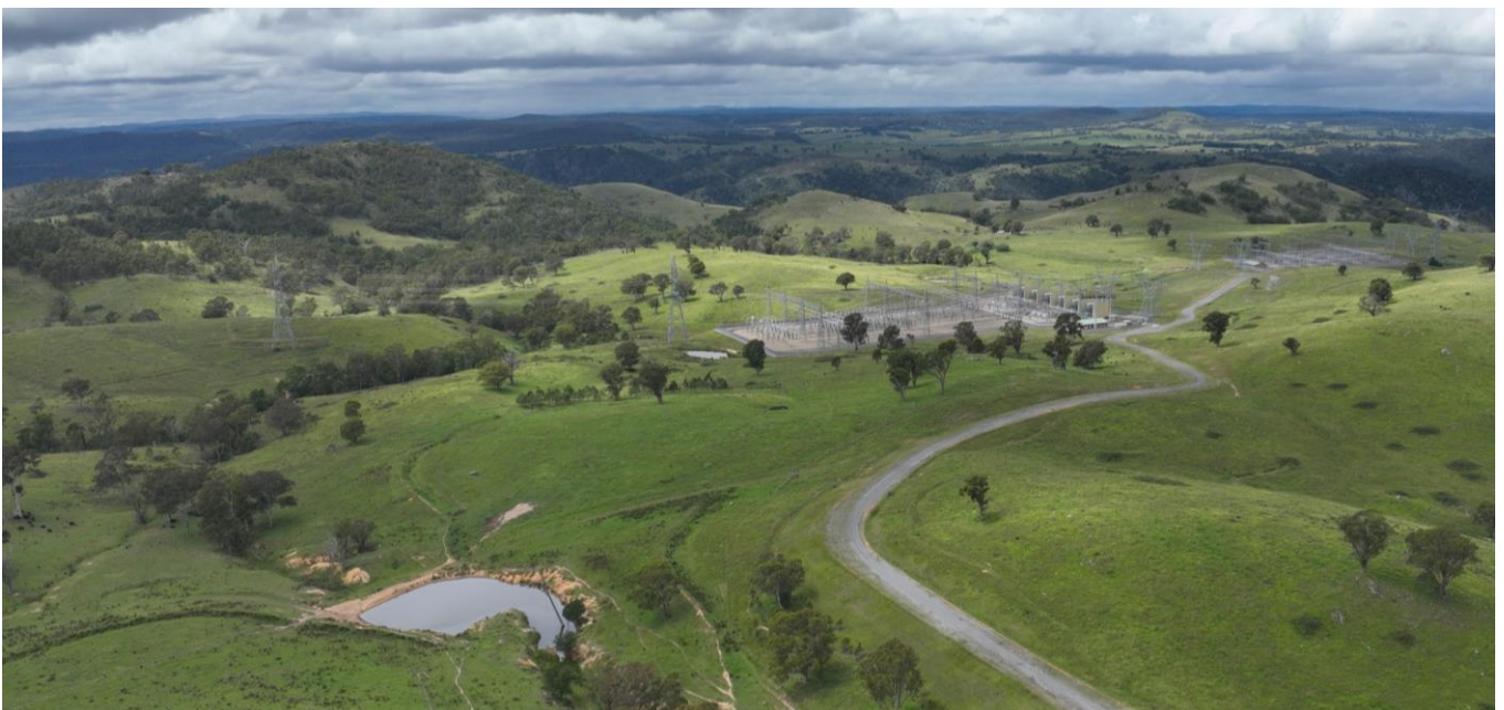
Aerial view of the existing Bannaby 500kV substation
