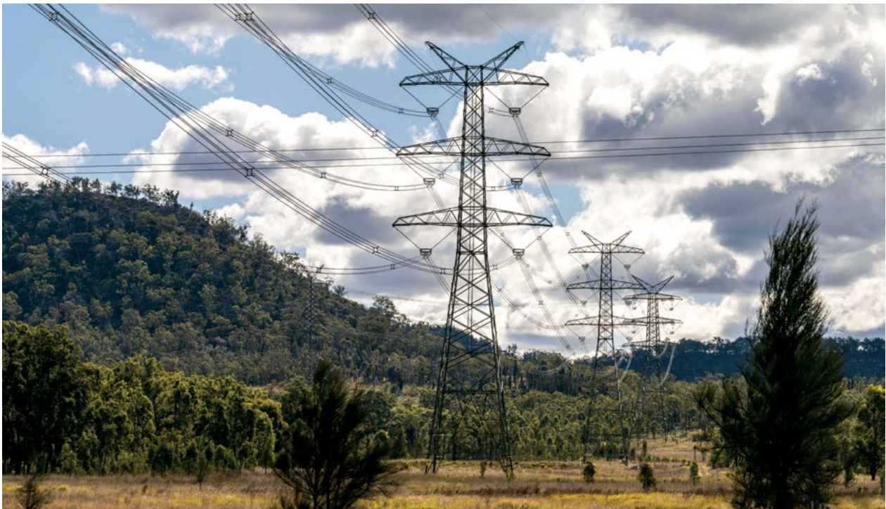
Pictured: 500 kV transmission towers in Muswellbrook, similar to those that will be built on HumeLink.
