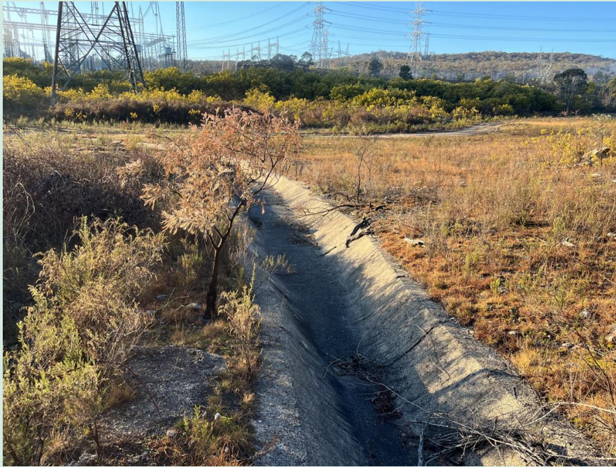
Concreted drainage line west of current substation, within heavily degraded and modified vegetation.
