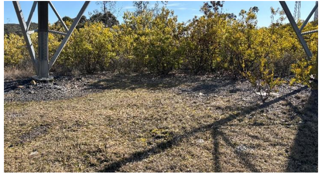
Plate 17: Typical ground surface cover at base of transmission tower within Subject Area
