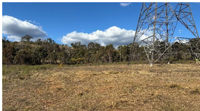
Plate 13: View east towards Structure 432, showing cleared easement area
