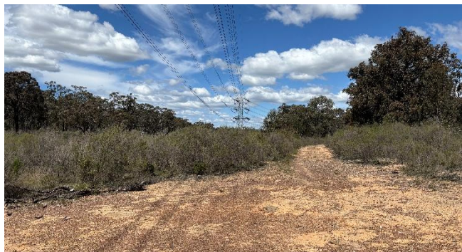
Plate 8: View south of easement towards Structure 356.
