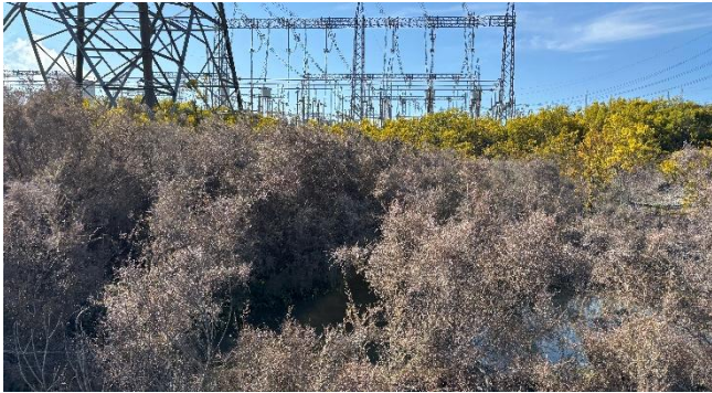
Plate 16: View east towards dense vegetation and substation complex
