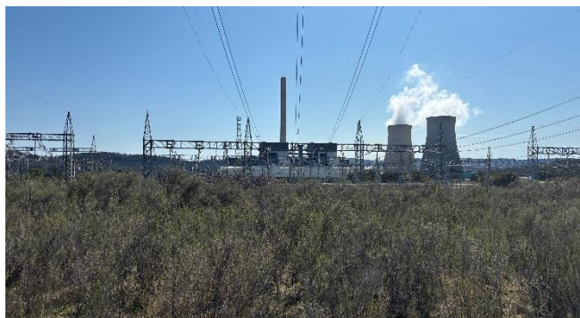
Plate 22: View north towards Substation complex
