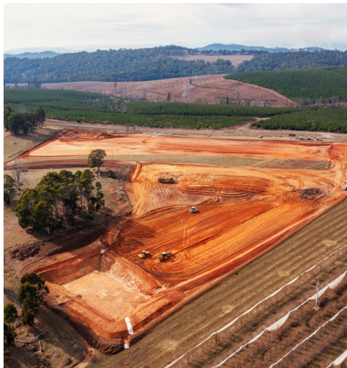
The Kunama worker accommodation site showing a water harvesting pond under construction.
