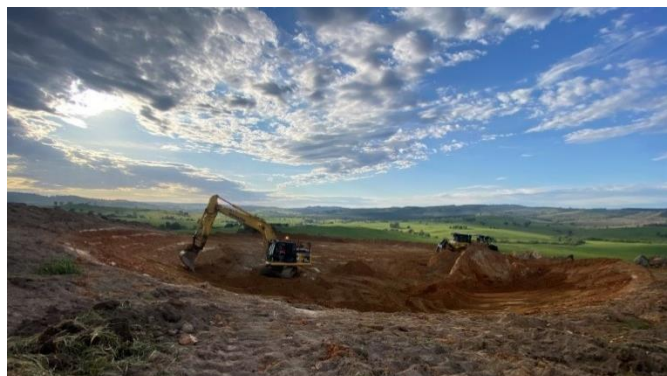
An excavator preparing a tower pad
