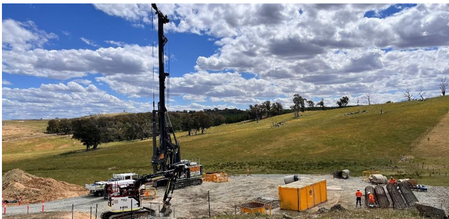
An example of a piling rig at work to drill foundations
