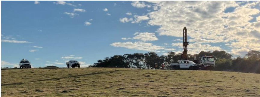
A geotechnical inspection being carried out near Bannister (May 2025)
