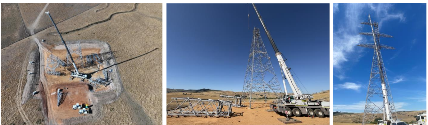
Examples of tower assembly and erection near Adjungbilly for HumeLink East
