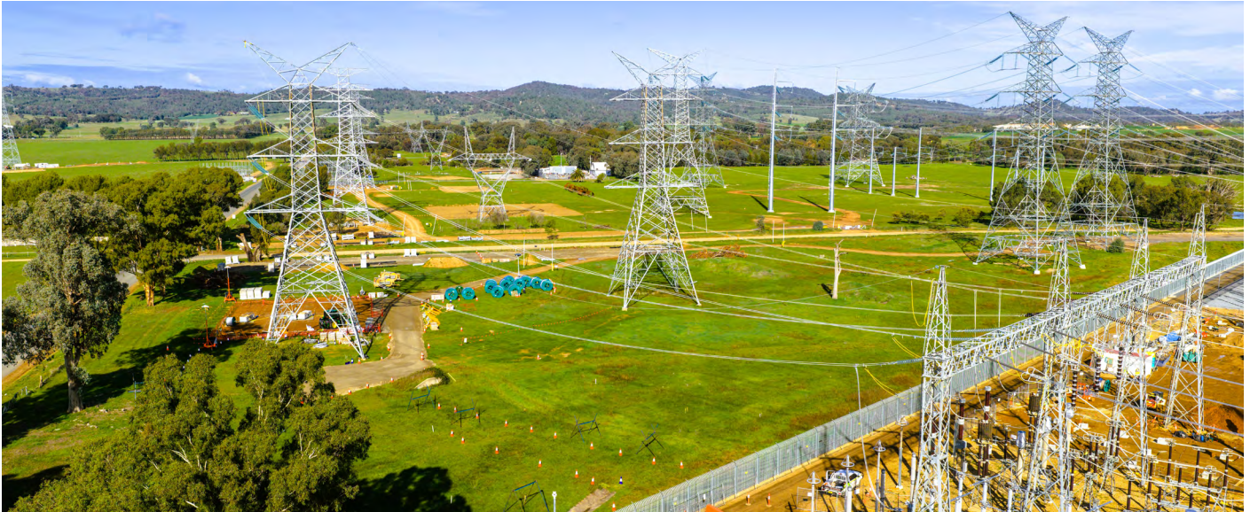
The first conductor cables have been installed on HumeLink West transmission towers leading into Wagga Wagga Substation.
