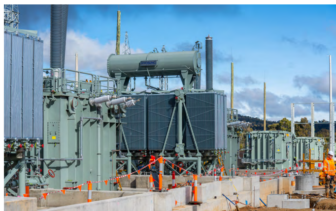
Both Maragle and Gugaa substations have received deliveries of electrical transformers and reactors via the Hume Highway and local roads from Port Kembla, with such shipments set to continue throughout July.
