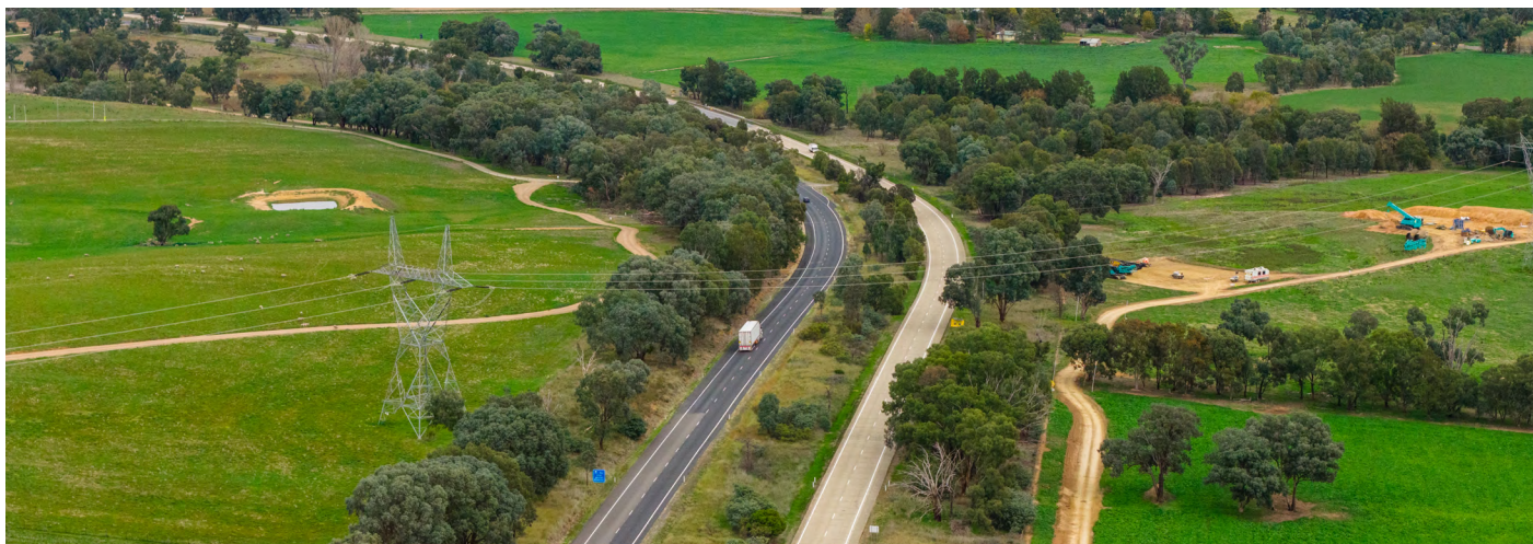
The crossing point of the Hume Highway at Keajura, south of Tarcutta, where scaffolding and netting is being installed to hurdle live traffic.
