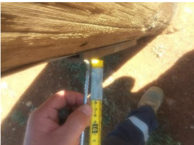
Figure 2-5 Measured hollow section at pole
