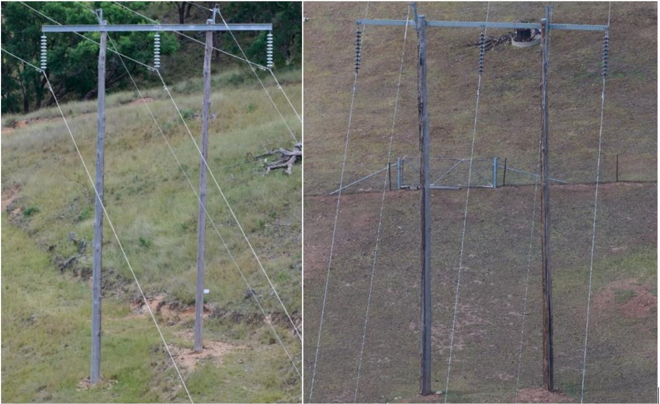
Figure 2-2 Wood pole structures on Line 94M.
