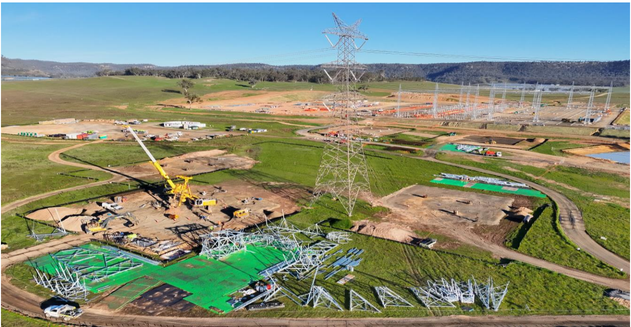
Aerial image of Transgrid/Zinfra Barigan Creek enabling works project site
