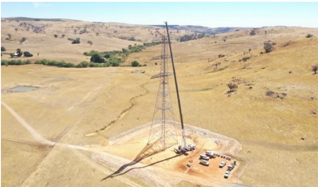
Tower erection began in December 2025 near Adjungbilly.
