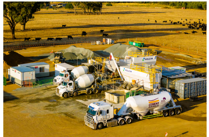
The Tarcutta batch plant will be decommissioned soon.
