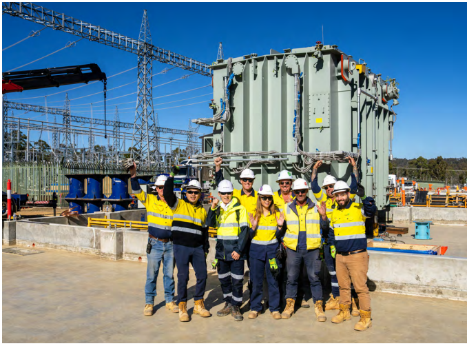
Workers celebrate successful delivery of another transformer at Maragle.
