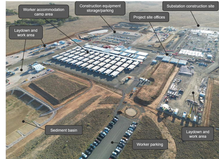
Example: Dinawan construction compound and accommodation camp, EnergyConnect (NSW – Eastern section) project
