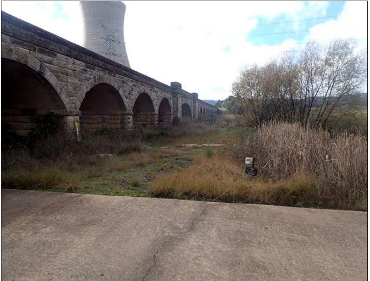
View east showing the Wallerawang Rail Bridges over the Coss River.
