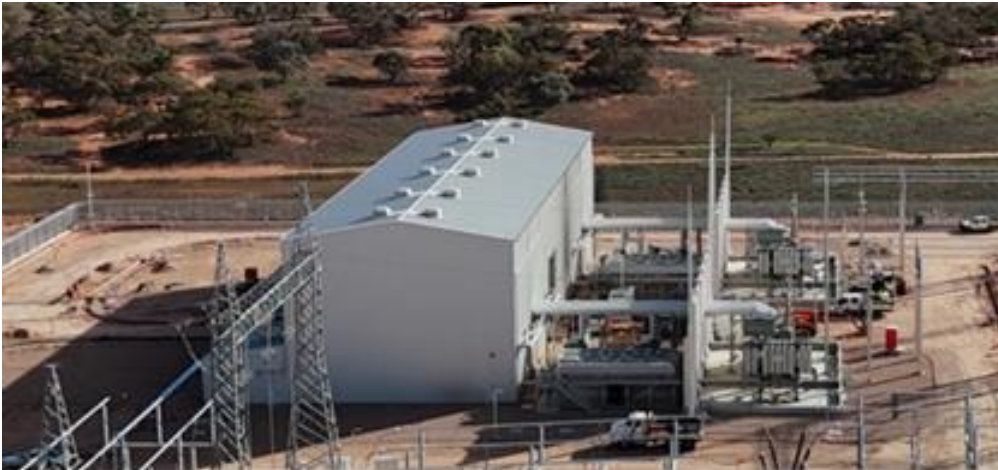
Figure 2-1 Photograph of a syncon housed within a building (example only)
