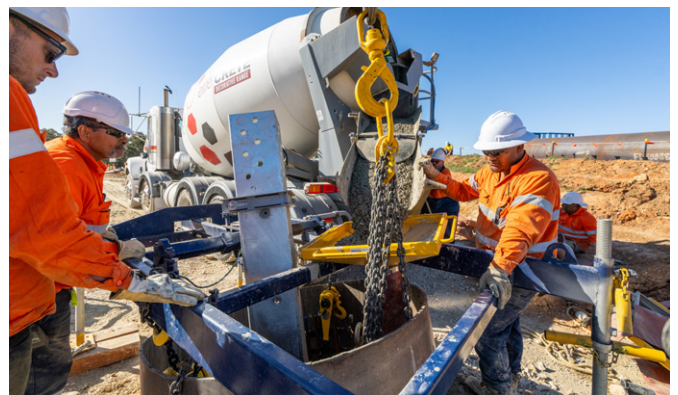
Figure 5: HumeLink first tower foundation construction.
