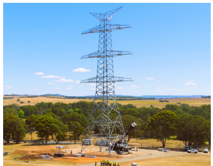
Figure 1: HumeLink West non-alpine 500 kV transmission tower ready for stringing.
