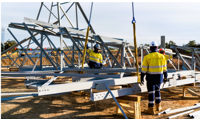
Figure 4: HumeLink West transmission tower under assembly south-east of Wagga Wagga.
