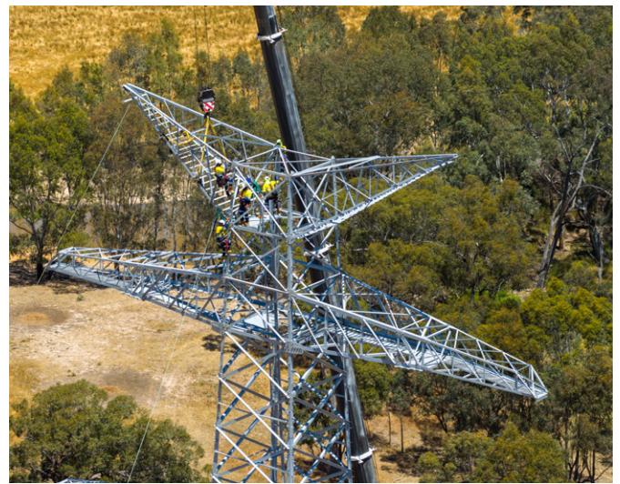
Figure 6: HumeLink tower erection underway south-east of Wagga Wagga.
