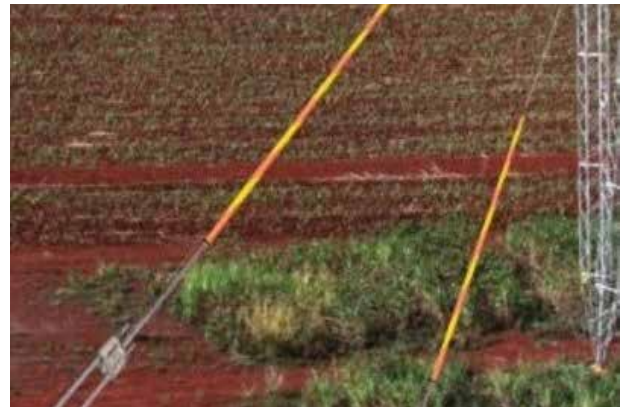
Reflective sleeves on a guyed tower
