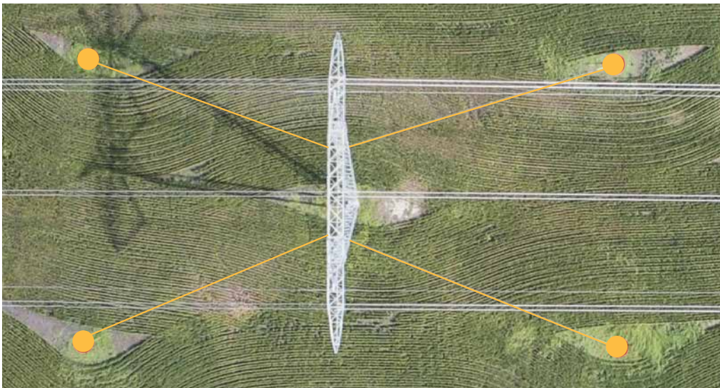
Farming operation with guyed tower installed (navigating between guy wires and centre mast). Yellow dots identify guy attachment locations.
