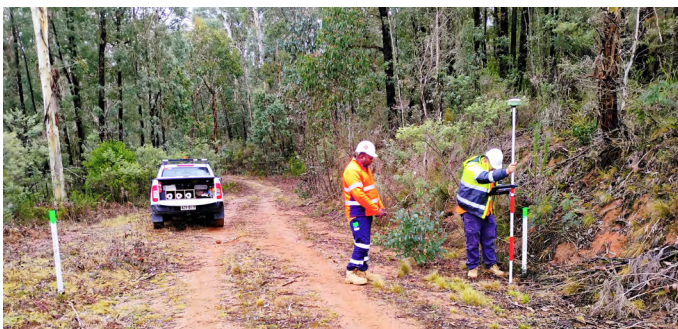
Local surveyors check levels for upgrade of an access track.
