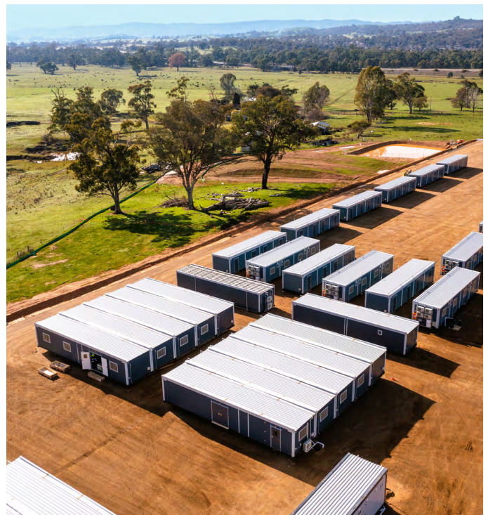
Temporary prefabricated modular building units being installed at Tarcutta.
