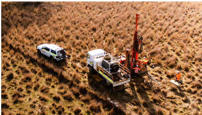
Specialist contractors set-up the drilling rig at each transmission tower site.
