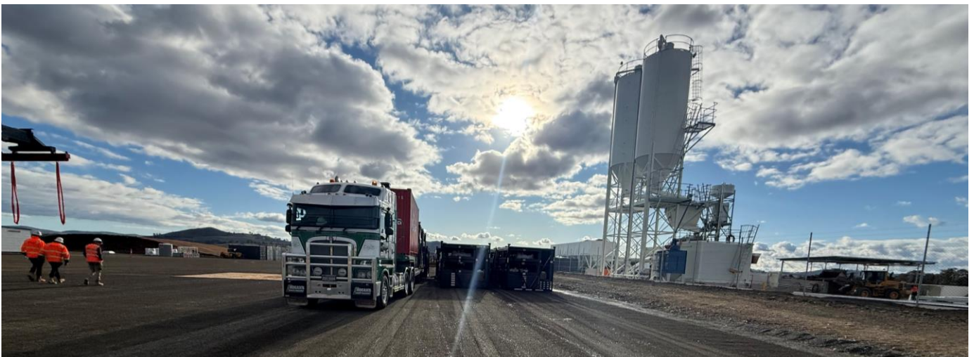
A truck delivering containers to the Yass Worker Accommodation Facility (July 2025)
