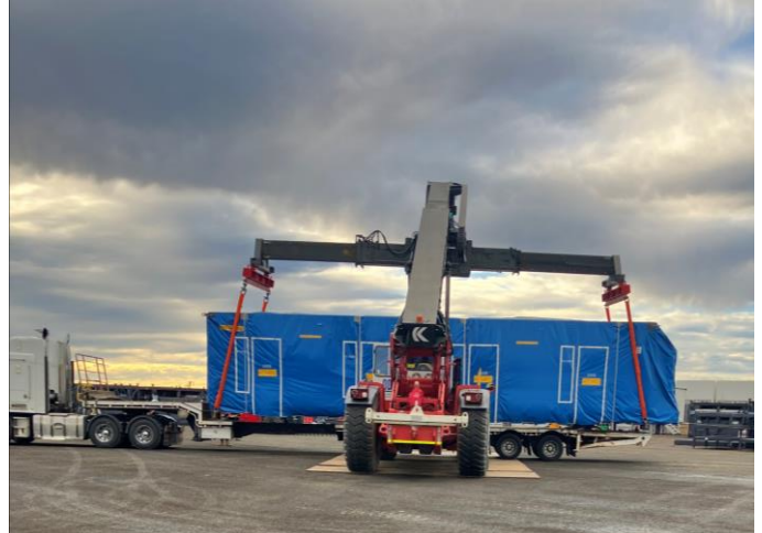
The first modular buildings being delivered to site (July 2025)
