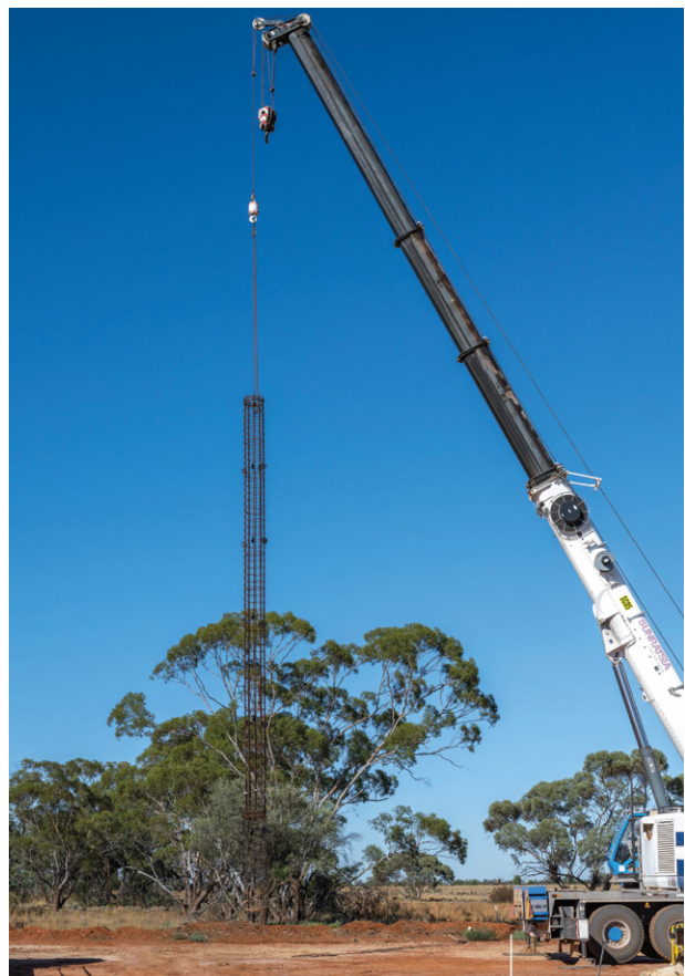
Pictured: A crane manoeuvring materials onsite.
