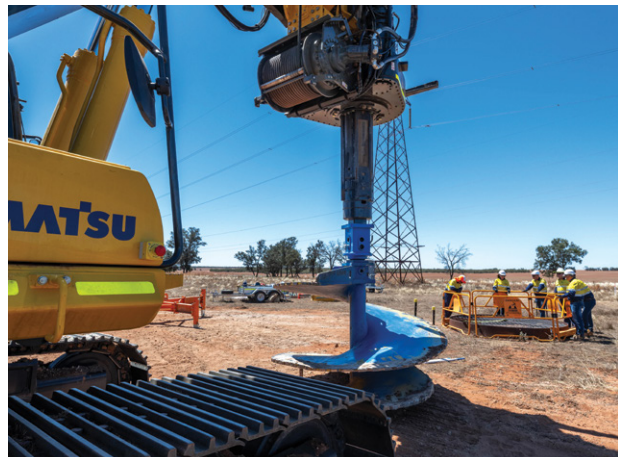
Pictured: A drill preparing transmission tower foundations.
