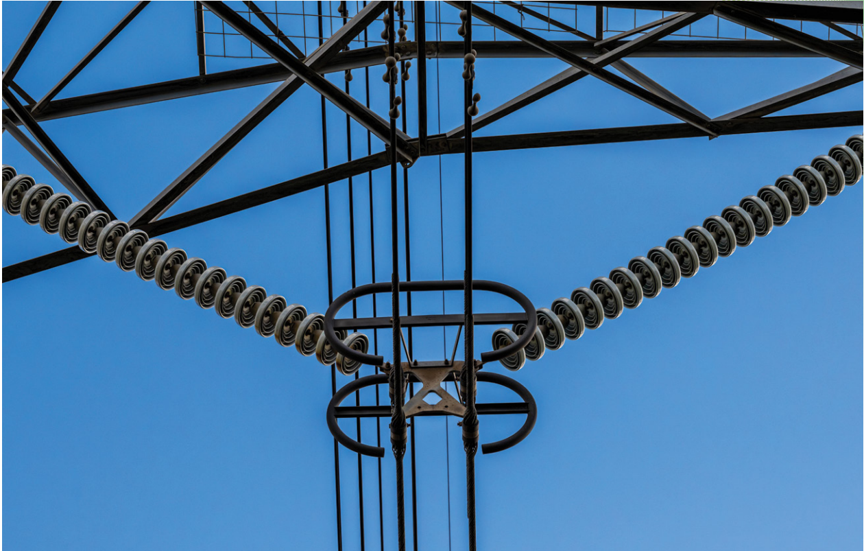
Pictured: Corona rings also known as 'grading rings' help reduce noise, providing a smooth surface around sharp edges, such as bolts and connection pins.
