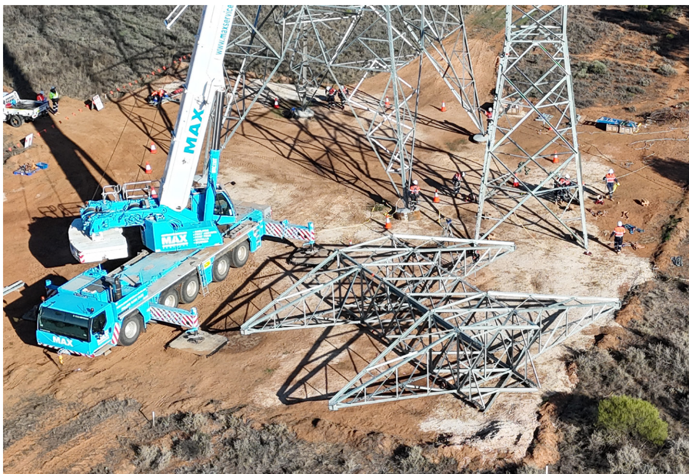
Figure 6: Tower assembly and erection on Project EnergyConnect.
