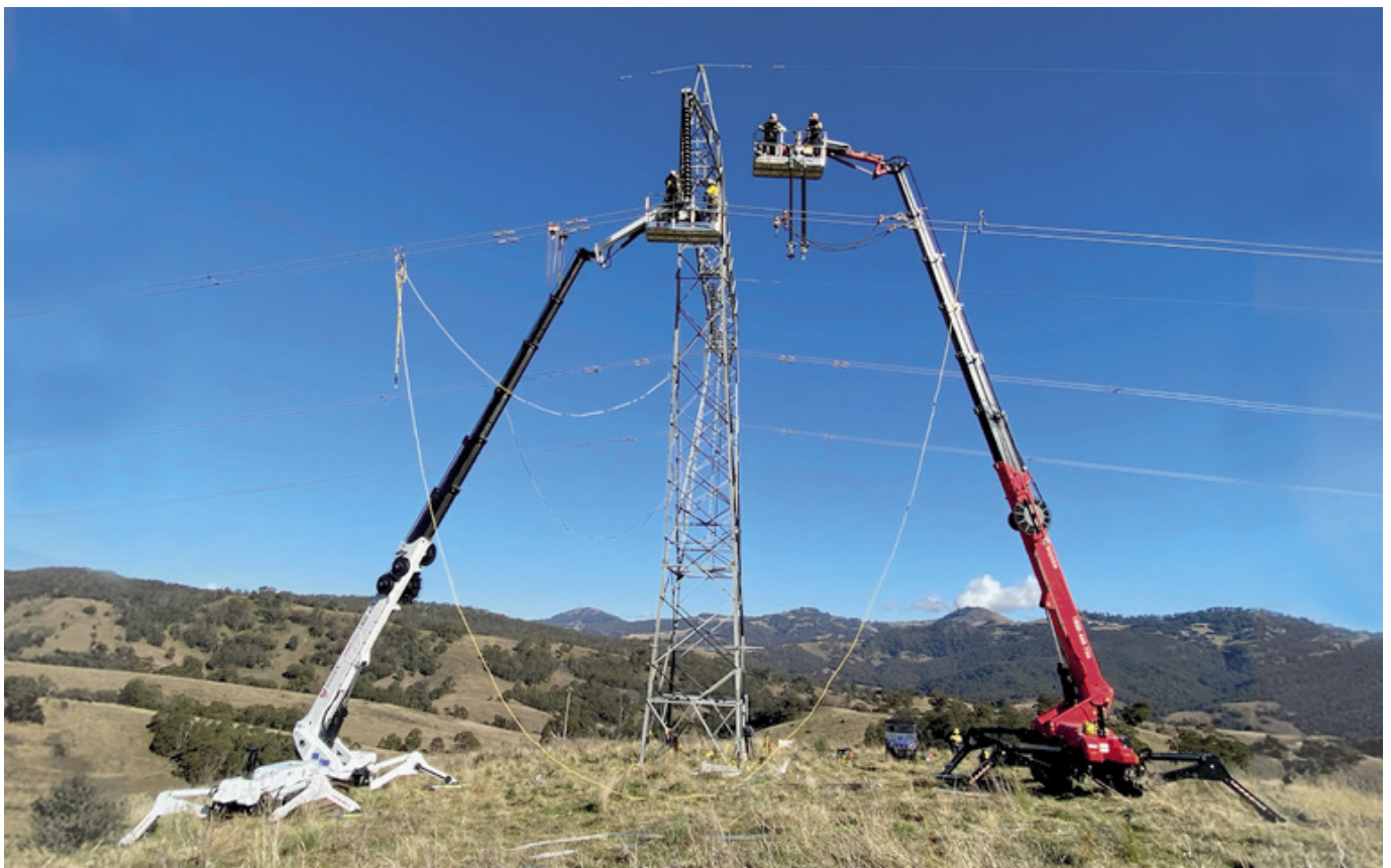
Figure 2: Two 500 kV transmission towers being assembled on a Transgrid site.
