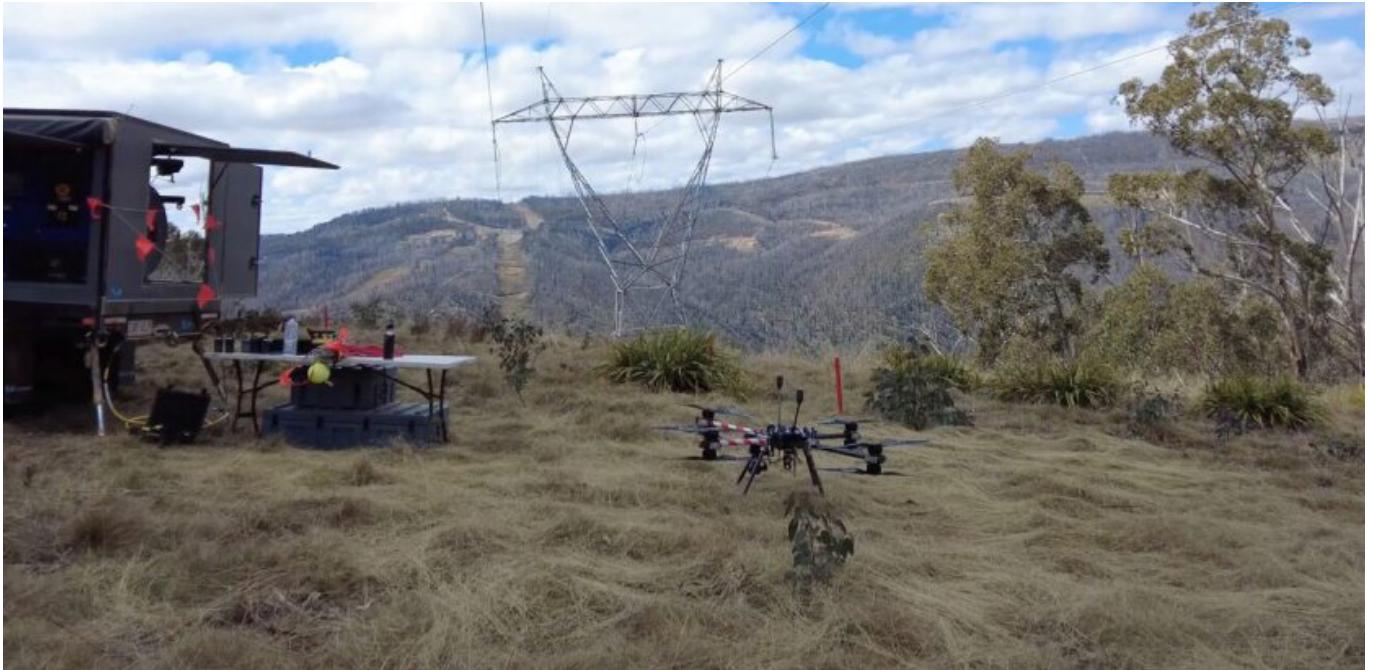
Figure 8: Example of drone stringing system.
