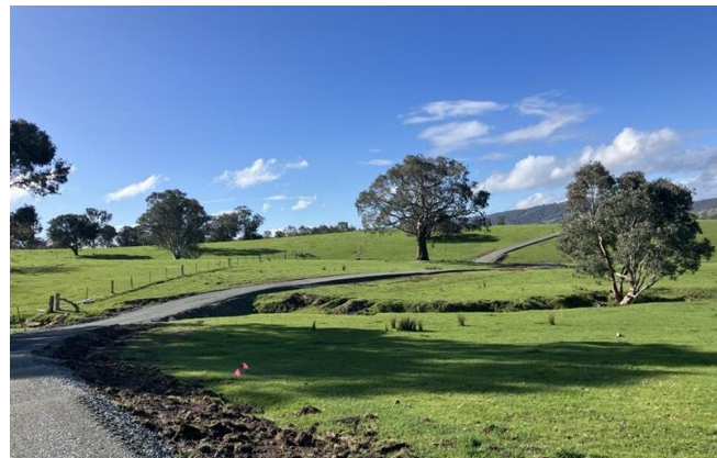
An example of an access track for HumeLink East
