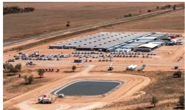
Pictured: Water storage pond located near construction worker accommodation at Project Energy Connect west of Wagga Wagga.
