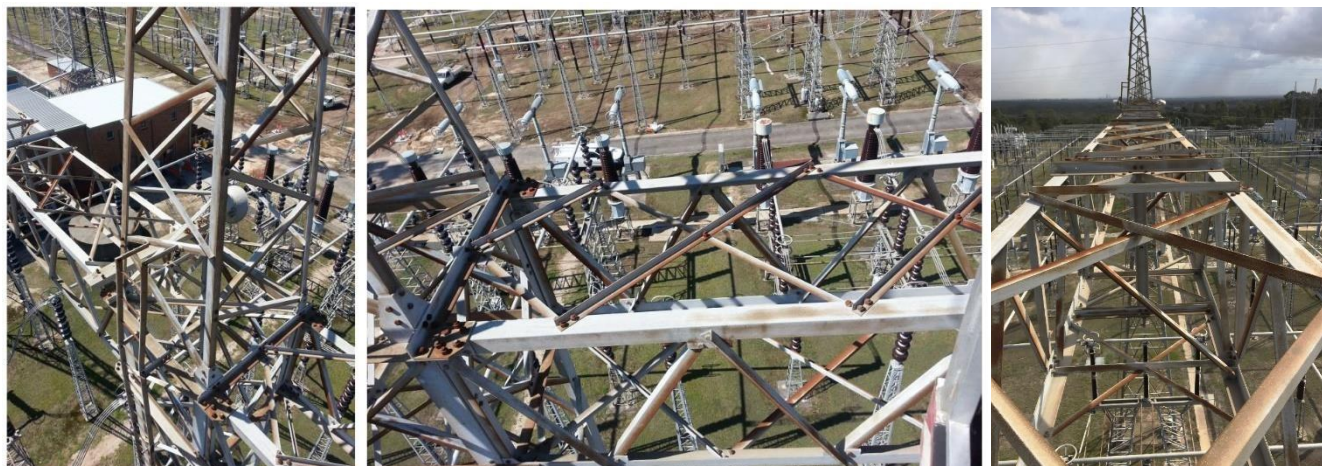
Figure 2-3 Typical gantry steel members showing corrosion
