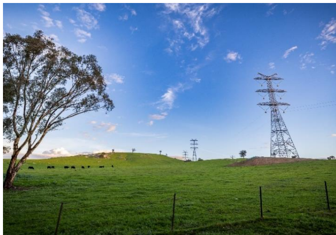
Completed towers near Adjungbilly
