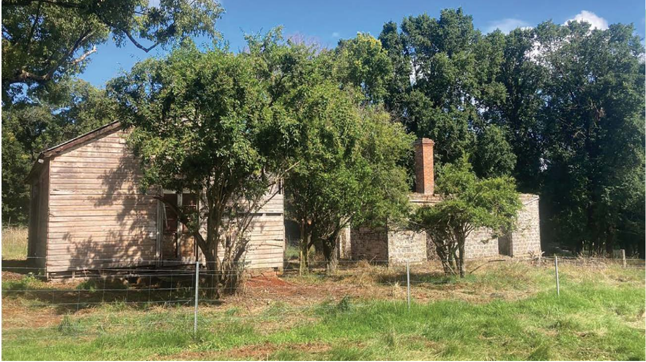
Pictured: Kiley's Run located two kilometres west of Adjungbilly, at least 200 metres west of the project footprint. (Image supplied by Forestry Corporation of NSW)
