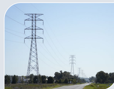
Figure 2: Example of a free-standing 330 kV transmission line structure.
