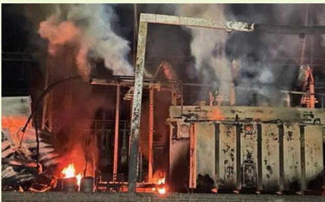
Left: Dapto transformer failure June 2022.
