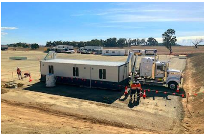
An accommodation module being delivered to the site.
