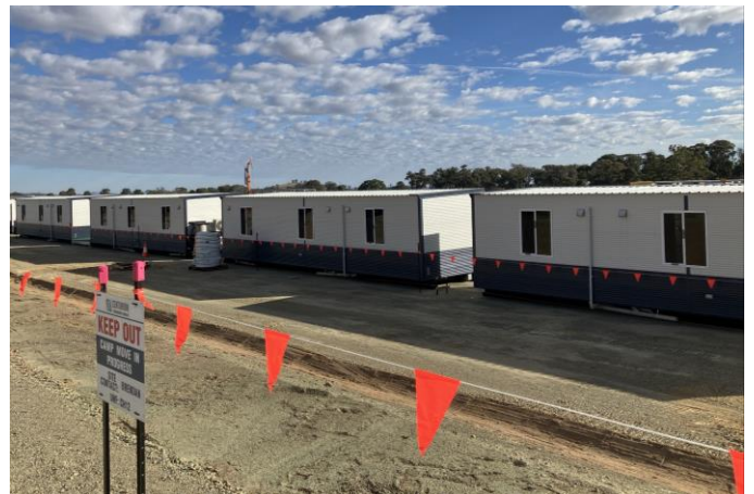
Accommodation modules in place at Adjungbilly.
