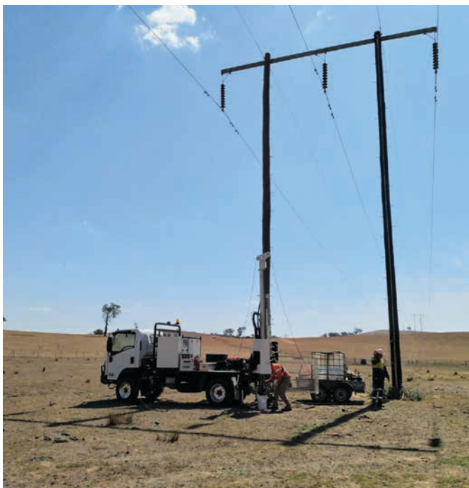
Truck-mount borehole drill rig on site
